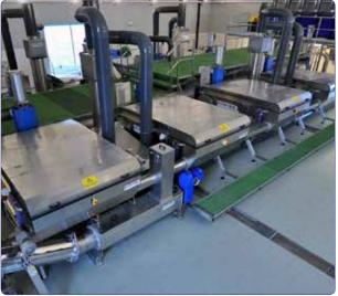
For those expanding primary or secondary capacity where land is expensive or unavailable, a Salsnes Filter system is ideal. It will typically use  $1/10^{th}$  the land of conventional treatment systems. The wastewater treatment plant in Tromso, Norway would have needed 21,530 ft² (2000 m²) of land to install clarifiers. Instead they installed a Salsnes Filter system and only used 1,600 ft² (150 m²) of land.
