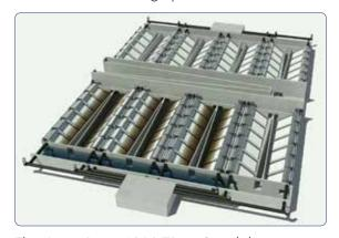
The Agua Prieta WWVTP in Guadalajara Mexico arranged modules to treat 350 MGD (1325 MLD) of stormwater using only 10,550 ft² (980 m²) of land. Primary settling tanks would have needed 215,000 ft² (20,000 m²) of land.
